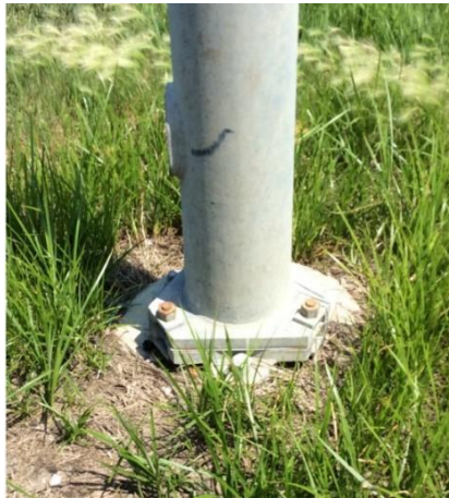
Good – some wear but structurally sound
