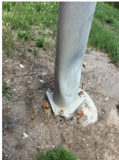
Very Poor – Serious deterioration/damage – fix as soon as possible
