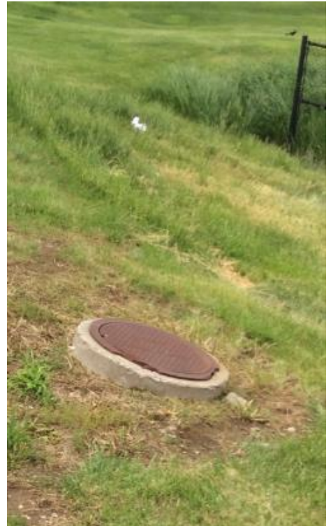
Good – some wear, but structurally sound
