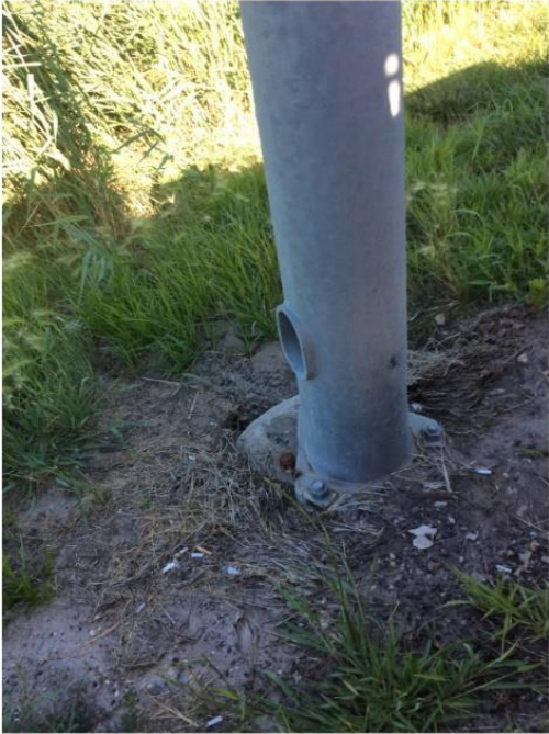
Door missing or damaged
